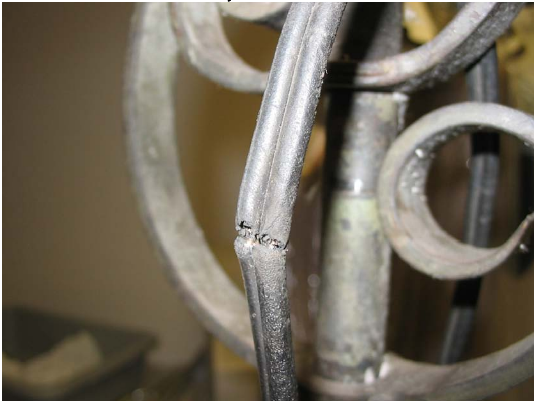
F2 – Defective cord caused by misuse that later arced and caused a fire
