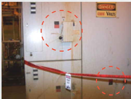
Figure 2: The highlight at the top left shows the racking handle for the R1 starter. The highlight at the bottom right shows the racking handle for the Q101 ("M" starter).
