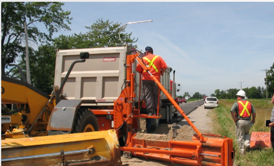
Figure 1: The dump truck/grader combination device working on the shoulder of the road.
