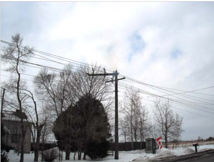
Image 8: 'Before' photo of pole fire
