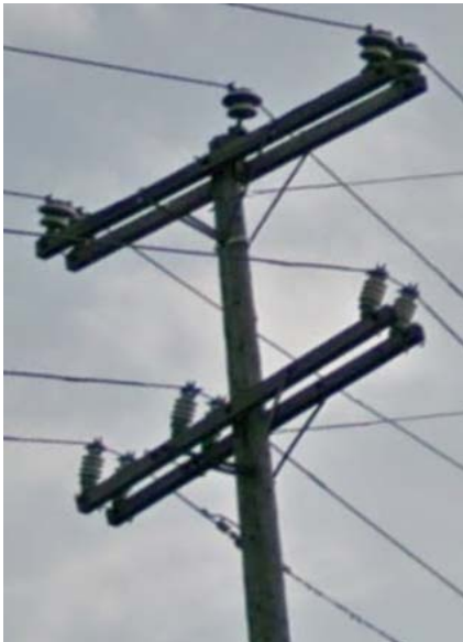
Image 6: Double Crossarm Configuration
