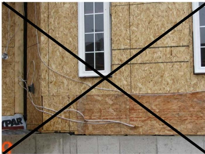
The intent of this direction is to accommodate very short cable runs to specific exterior outlets. The wiring method cannot be used for wiring between or to interior outlets.
