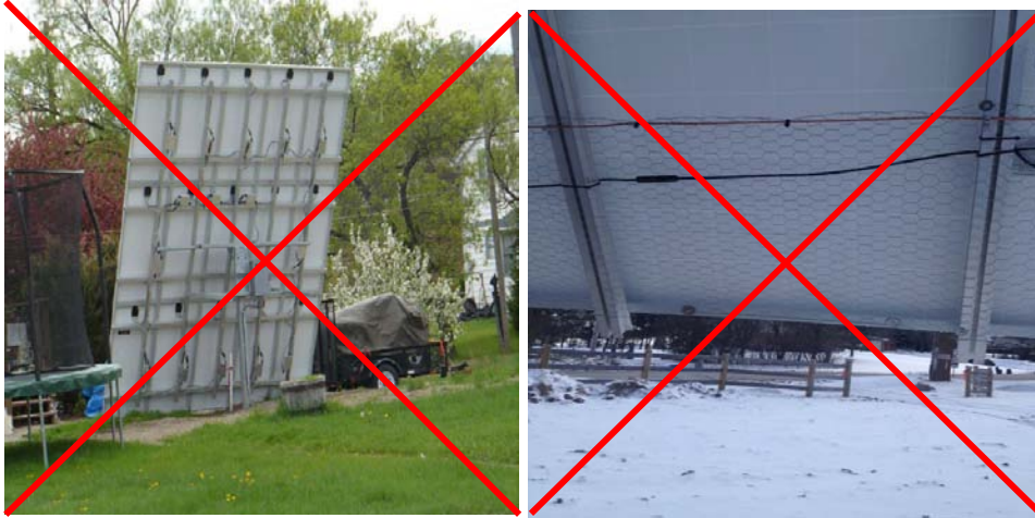
Photo B6 – example of using physical barrier around wiring
