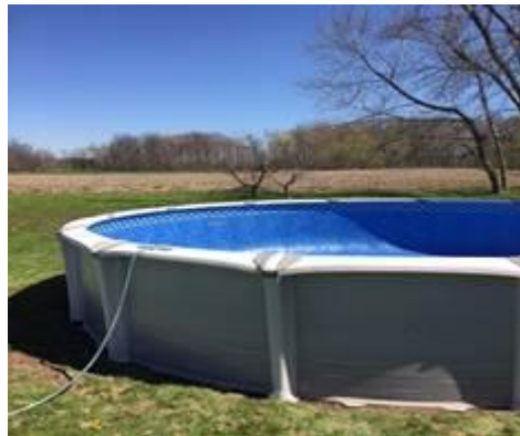
Photo B2 – Above ground pool with non-conductive supports
