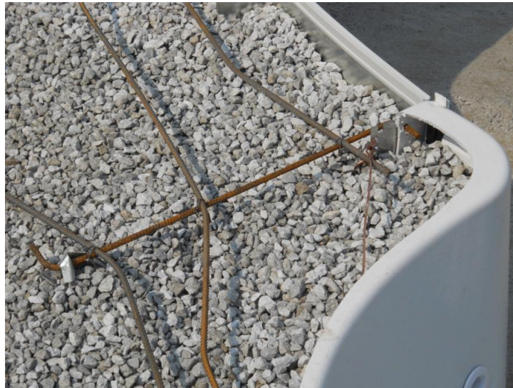
Photo B5 – A conductive mesh below the deck in solid contact with the pool
