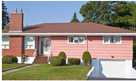
ESA streamlined its ElecCheck service to focus efforts that address the aging infrastructure harm. Homes built prior to 1976 are at an increased risk of electrical fire and shock.
