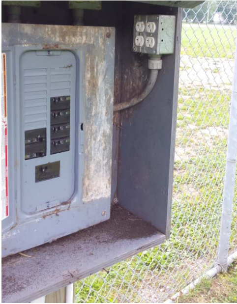
Photo F3 – Accessible and Deteriorated Enclosure
