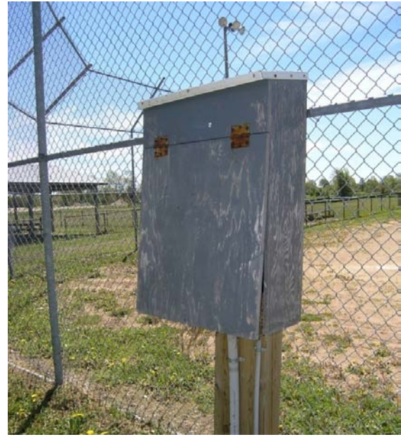
Photo F3 – Accessible and Deteriorated Enclosure
