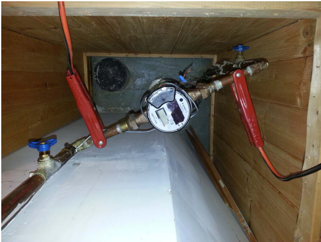
Photo B1 – Using automotive battery cables for temporary grounding jumper
