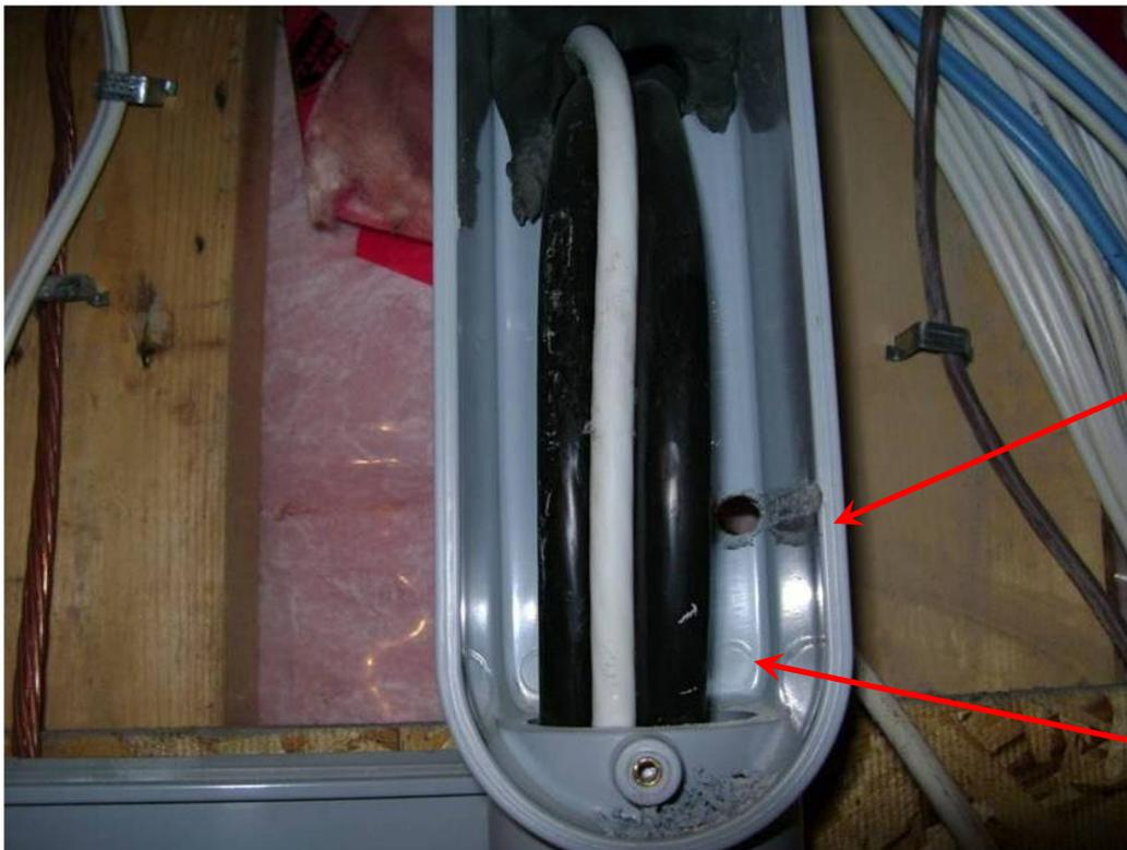
A Cable installer drilled a hole through the wall from the outside, without realizing the hole penetrated into the electrical conduit fitting and almost interacted with the energized wire.
