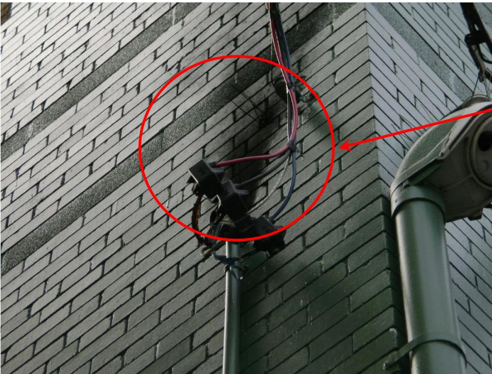
The arc flash went up the conduit and exited at the top of the mast. The arc flash also entered into the building and burnt out the service switch and meter base.
