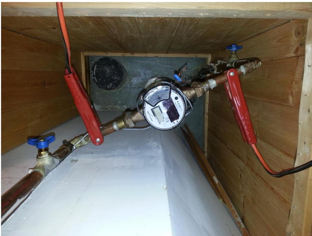
**Replacement water meter of the non-conductive type**
